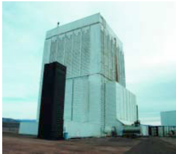
Building Structure that houses the dryers.
